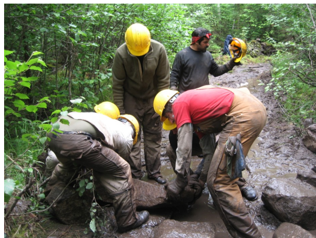
Participants work with their Foreman to repair a portage trail.
